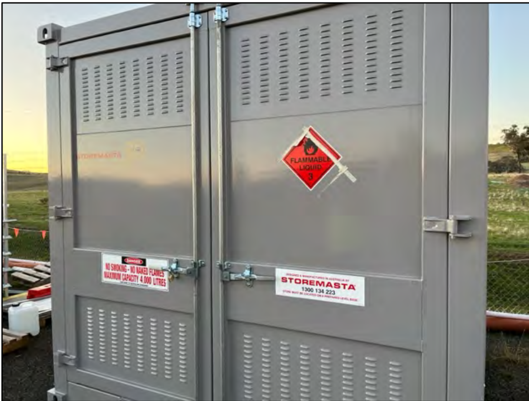
Plate 11: View of a bunded Dangerous Good storage container within the main site compound area.
