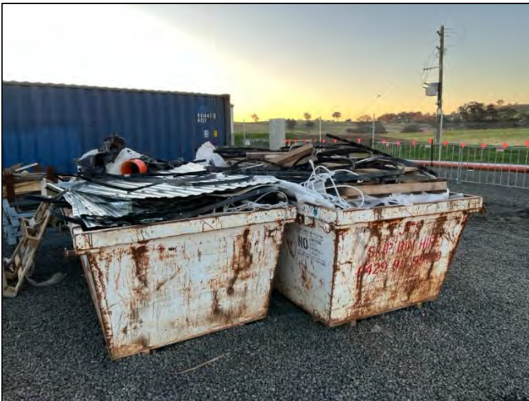
Plate 10: View of waste skip bins within the main site compound. While evidence of waste segregation was noted at some locations, in several instances overfilling of bins and comingling of wastes was also observed. It was noted, however, that housekeeping was generally of a good standard across the broader area of the site.
