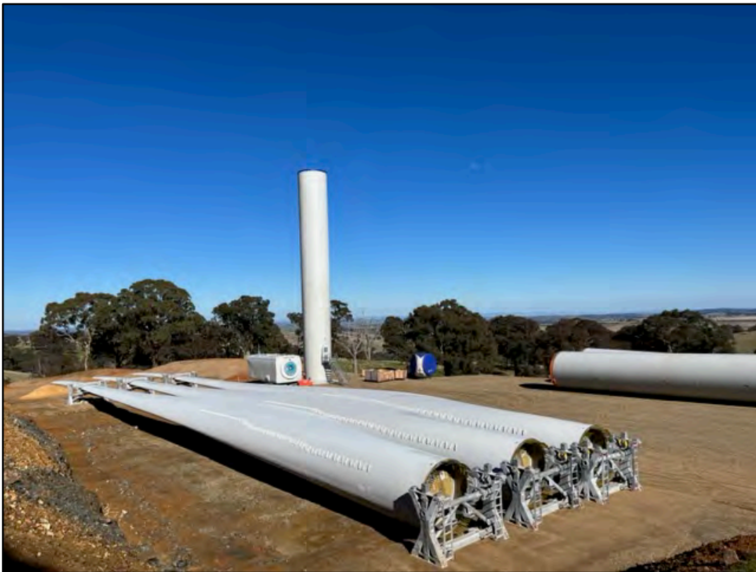
Plate 9: View of typical turbine infrastructure including supporting pier, generation nacelle and blades. This infrastructure was noted to be of low-reflectivity and an off-white colour.
