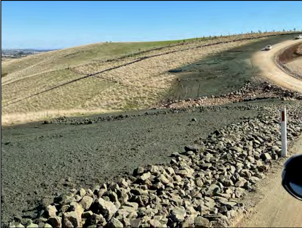
Plate 7: View of recently hydro-mulched work areas within the CG3 site. The application of hydro-mulch was noted to be of good thickness and coverage.
