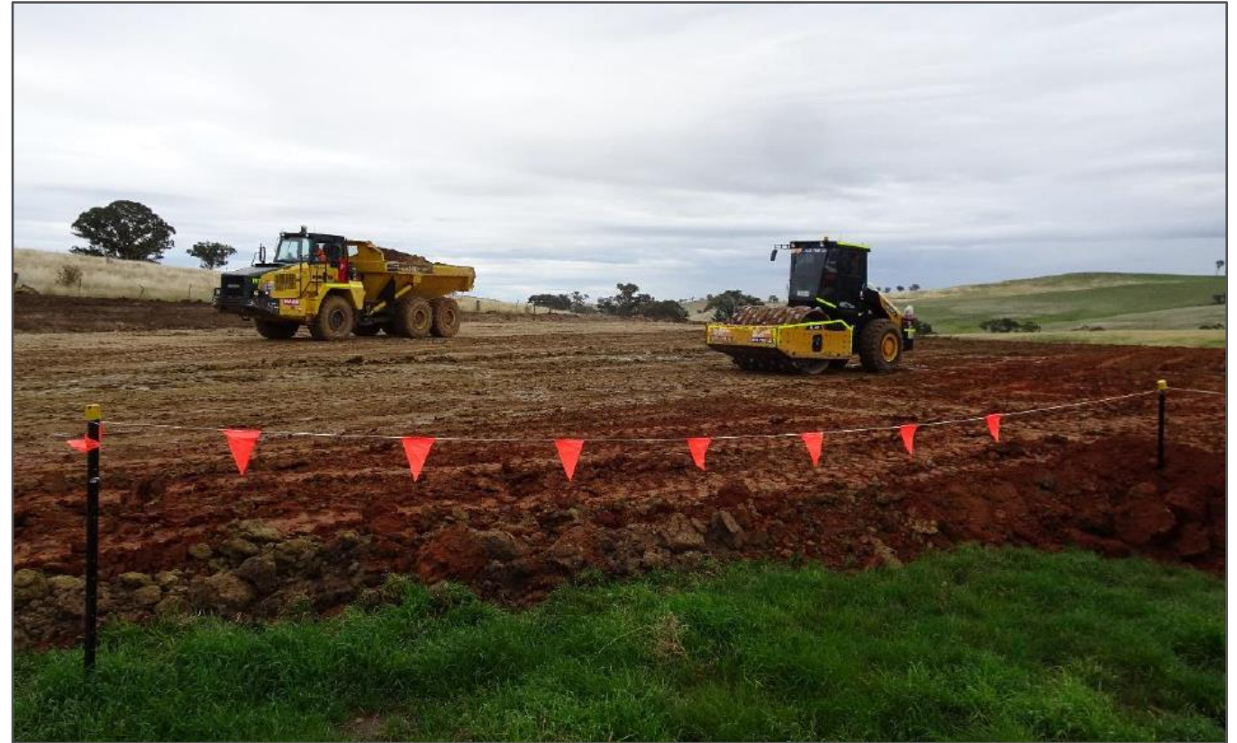
Earthworks for the temporary construction compound pad
