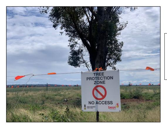
Plate 4: View of sensitive area protection signage and fencing installed in accordance with Development Consent biodiversity and heritage management conditions.
